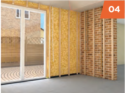
04 The interior has services added and is battened ready for internal finish.
