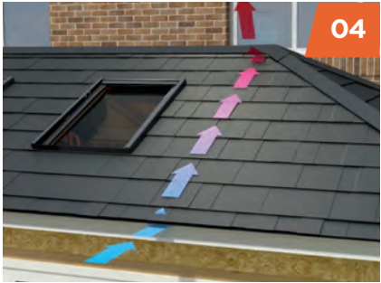
04 Roof is battened and chosen tile is added ensuring weather-tightness. The gutter and external trim are secured.
